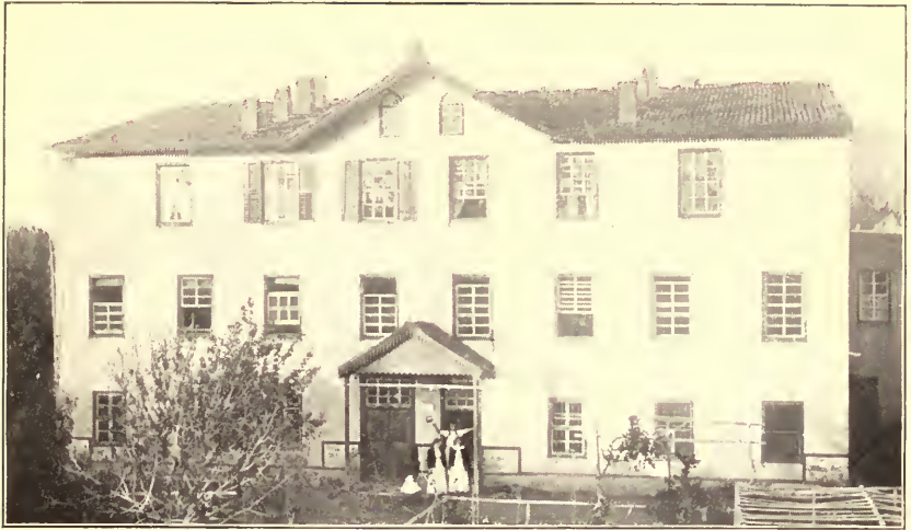
THE HOSPITAL AT VAN
